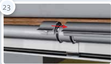
Connecting with deflector coupling
