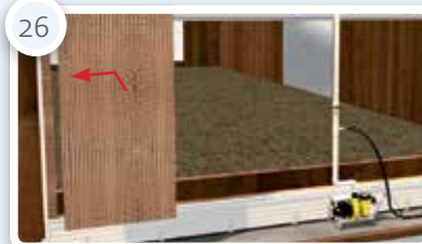
Setting in pads from left to right
