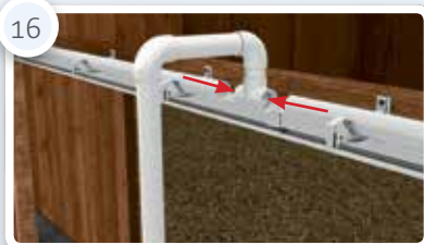
Setting of water distribution pipe
