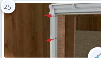
Setting and fixing pad end cover with 6 screws to wooden frame
