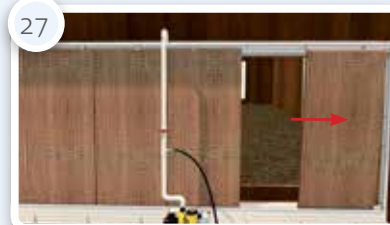
Setting next-to-last-pad on right
